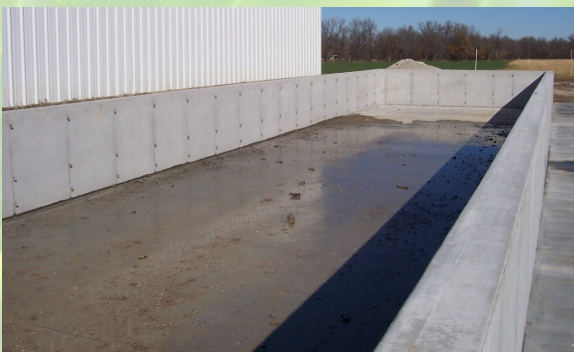
Containment for liquid fertilizer
